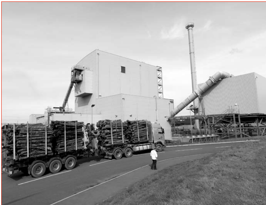
Western Wood Energy Plant at Port Talbot, Wales, generating 14 MW by burning 500 tons daily of wood and residues
